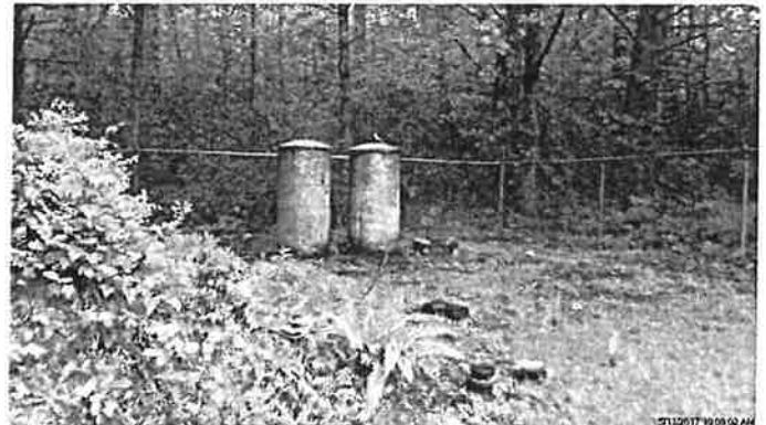
Inactive well #1 (S01) to the right of old hydropneumatic tank
