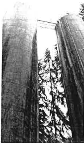
Catwalk between finished water reservoirs
